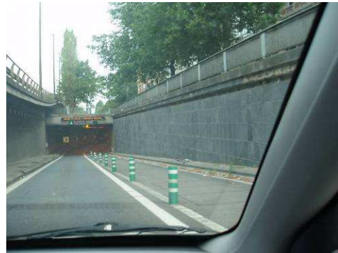
Tunnel Reyers-Meiser – affichage variable
